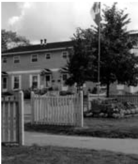
La Westridge Estates Housing Co-op à Charlottetown
